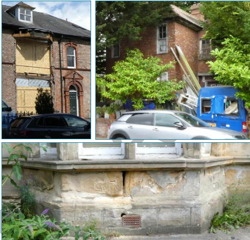
Top left 10, Polam Road with missing two storey bay window viewed from West Crescent. Top right 78, Woodland Road viewed from West Crescent. Bottom Disintegrating sandstone to bottom of bay window at [11] 67, Stanhope Road with remnants of a cement render which is likely to have caused/accelerated the decay. (Photos © Gaby Rose, June/July 2025)
